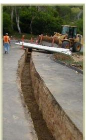
A: Typically, final pavement restoration will occur once the pipeline is installed, tested, and operational. For certain projects, temporary pavement or steel plates will need to be installed to maintain roadway service during construction. All pavement work will be completed in accordance with City of Solana Beach or County standards depending upon the location of the construction.
