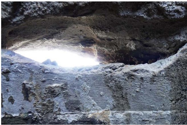
Close-up view of hole in Lake Hodes Dam
