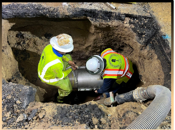
Staff installs pipe collar to repair break in large-diameter distribution pipeline.
