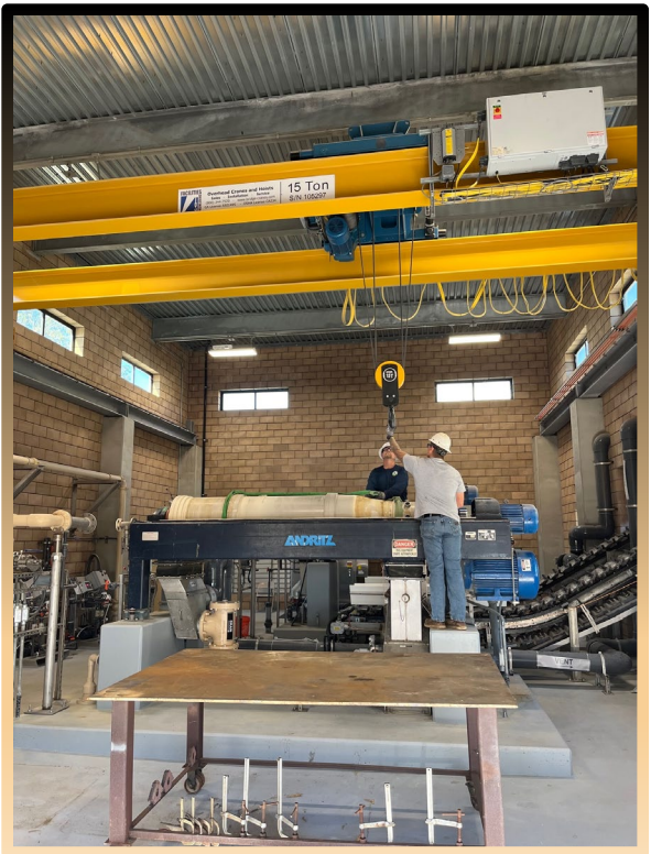
Staff repairs solids handling centrifuge at the RE Badger Treatment Plant
