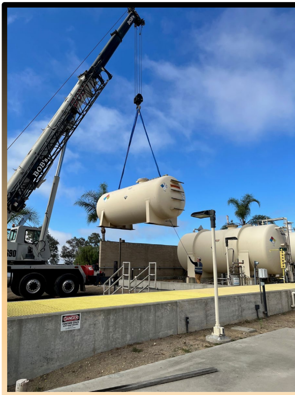
Staff installs new chemical process tank at RE Badger Treatment Plant
